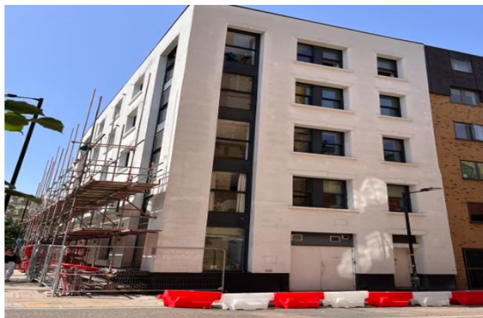
A photo showing Phase 1 Marshalsea Road Elevation scaffolding installation works progressing
